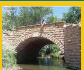
WPA Limestone Bridge at Denmark
